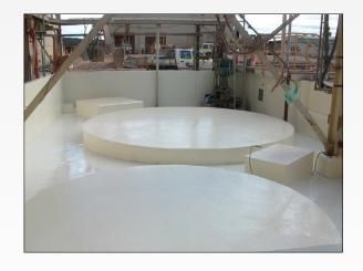
**Protective coatings** are another successesfull method of reducing negative effects on concrete. Recommendations of suitable coatings for the long term protection of concrete against these chemicals and other causes of damage, such as impact and abrasion, can be undertaken by Extrin. Specifications for the correct preparation and application of recommended coating products is also part of our expertise.
